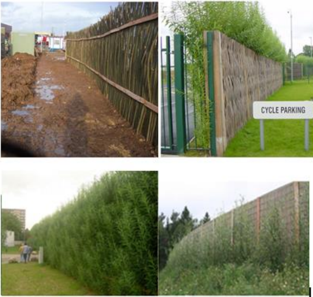
Figure 26: Examples of a living willow screen
